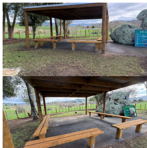
Photo: New shelter built replacing the previously covered signage.
